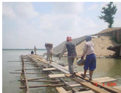
Fig.4e Slope footing enforcement
