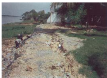
Fig.1a Gabion retaining wall
