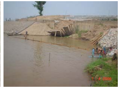
Fig.4d Slope rehabilitation works
