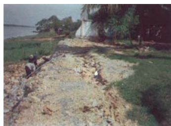
Fig.1a Gabion retaining wall
