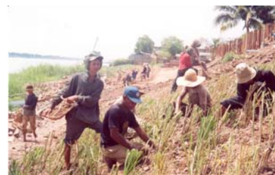
Fig.1b Embankment slope
