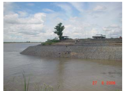
Fig.4f Man-made slope rehabilitation
