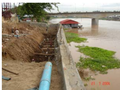
Fig.3a Retaining structure
