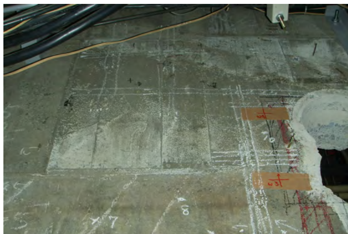
Fig. 5.23: Photograph of actual concrete wall to be surveyed
