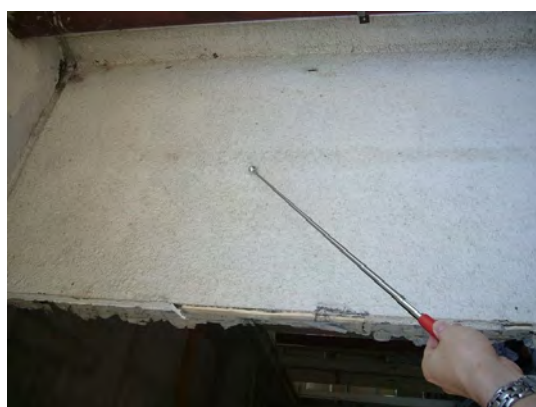
Fig. 5.2: Appearance of hammering test for debonding concrete wall
