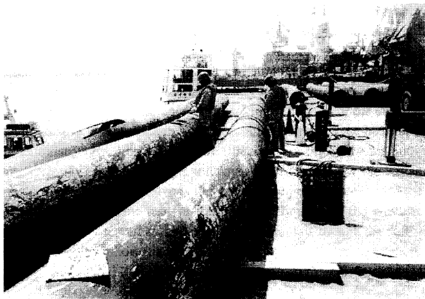
Figure 2.10: Failure of piles at Takahama (after Japan Association for Steel Pipe Piles, 1997)
