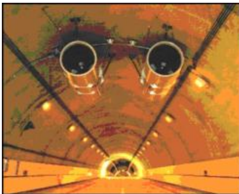
Fig. 1.29 Jet fan for tunnel ventilation system (1.48) .
