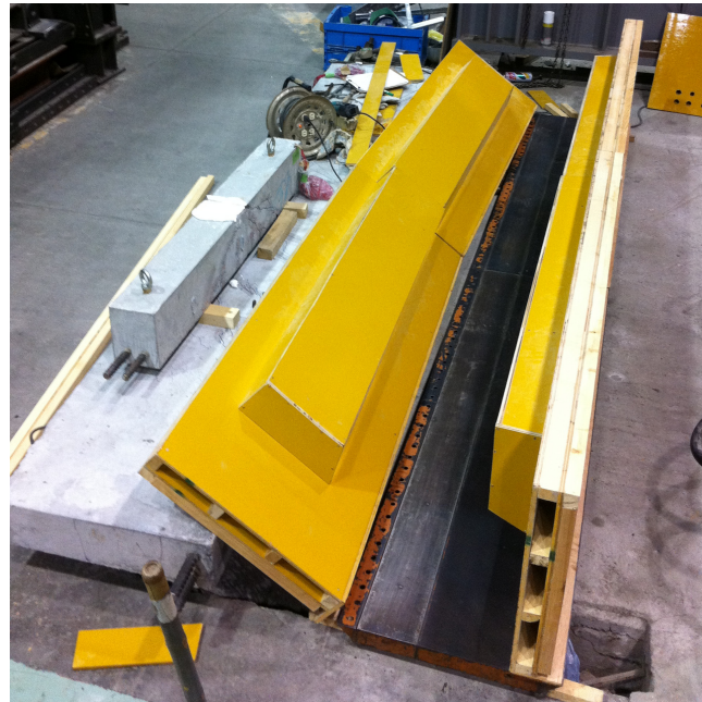
(b) Formworks for the specimens with d = 500 mm
