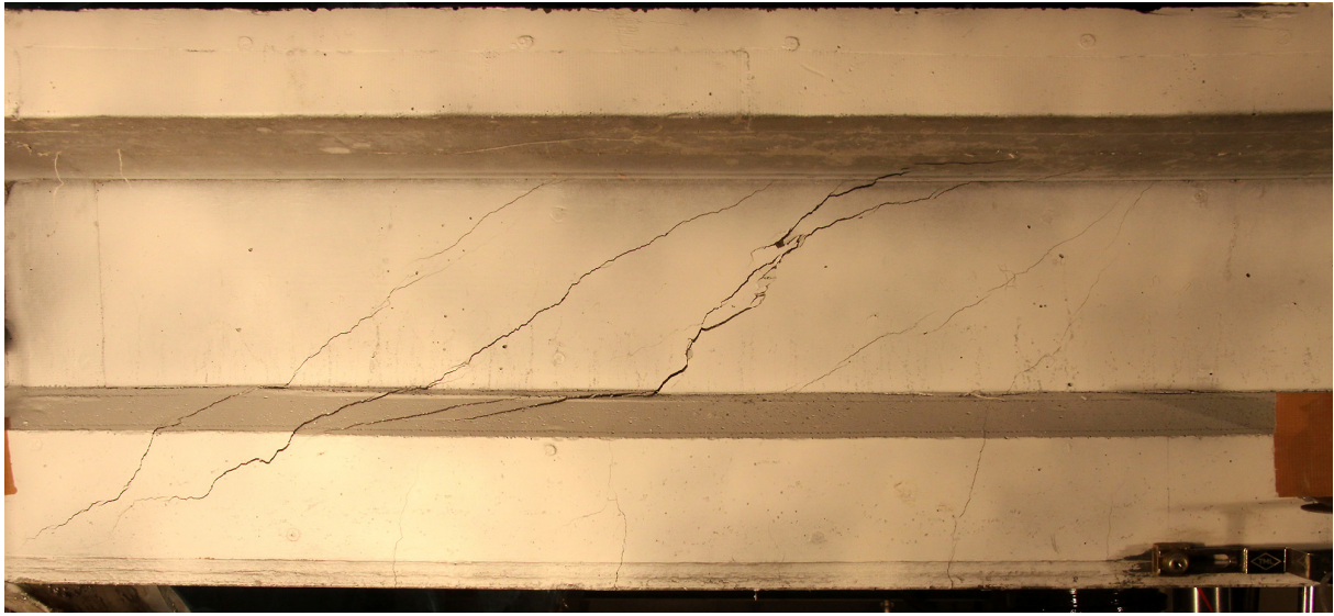
Crack pattern at the peak load: C-s150-I
