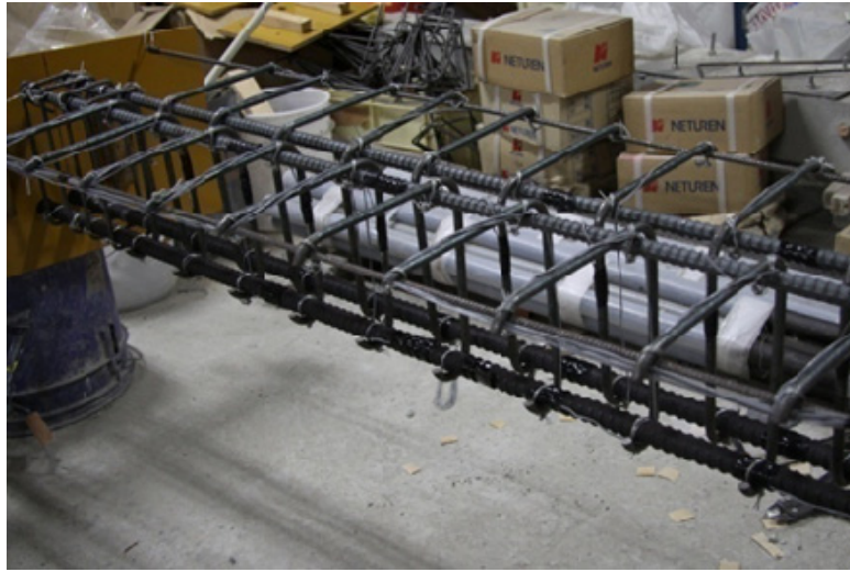
Photo 3-4 Steel bar cage for D-f500
