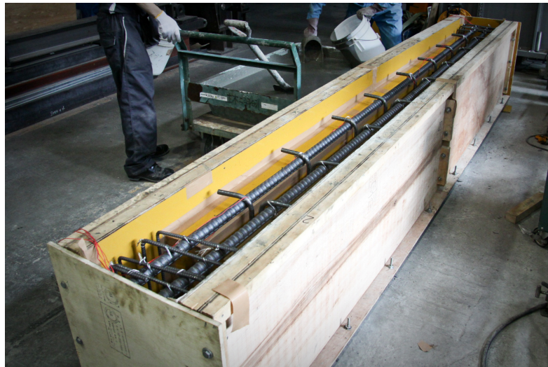
Photo 3-5 C-s370-II(16) ready to be casted
