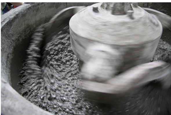
(5) Mixing mortar with coarse aggregate
