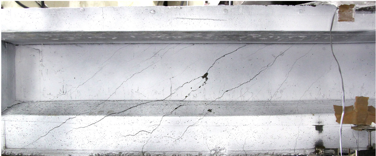
Crack pattern at the peak load: D-s90
