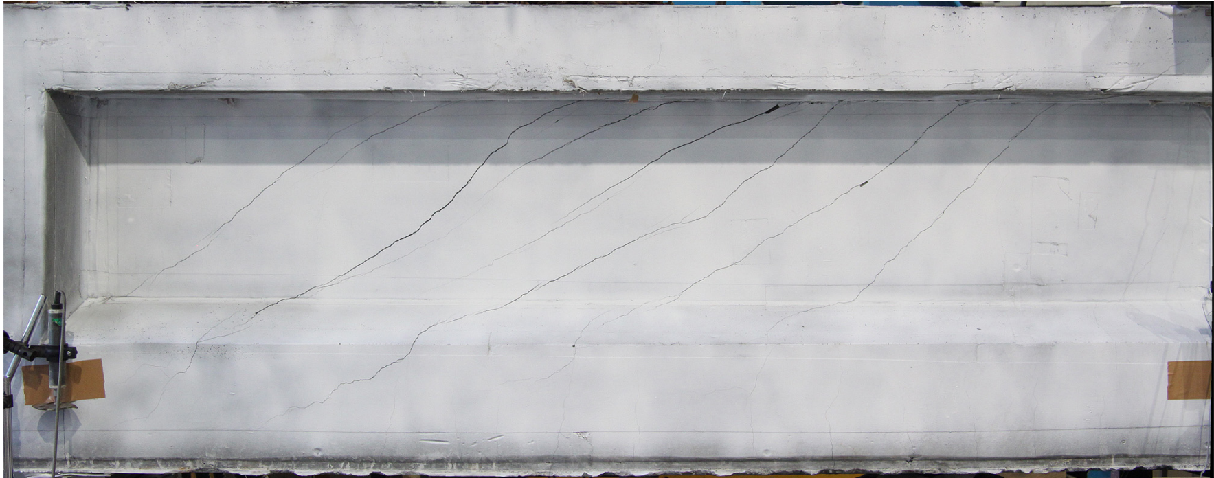
Crack pattern at the peak load: C-s230-I
