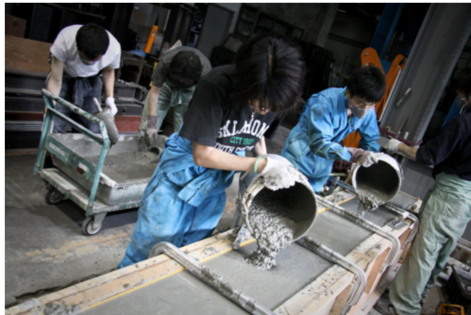
Photo 3-7 Casting self-compacting concrete
