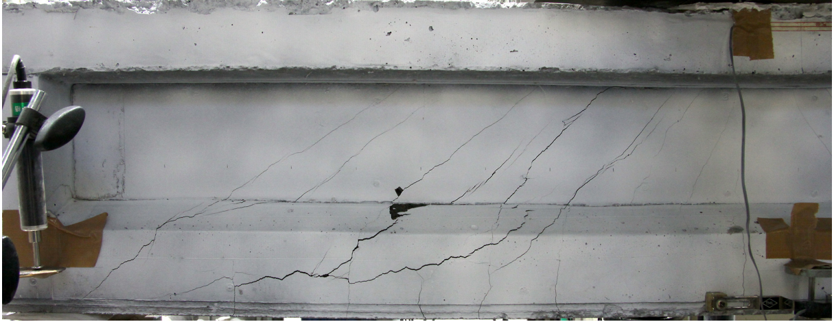
Crack pattern at the peak load: D-f150
