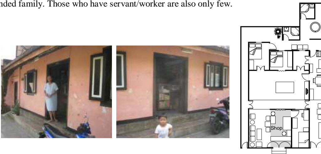
Figure 2.3. One of the Observed Javanese Shop houses
