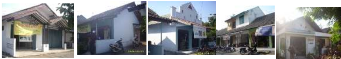
Figure 1.5. Recently Built Javanese Shop Houses (survey 2008)
