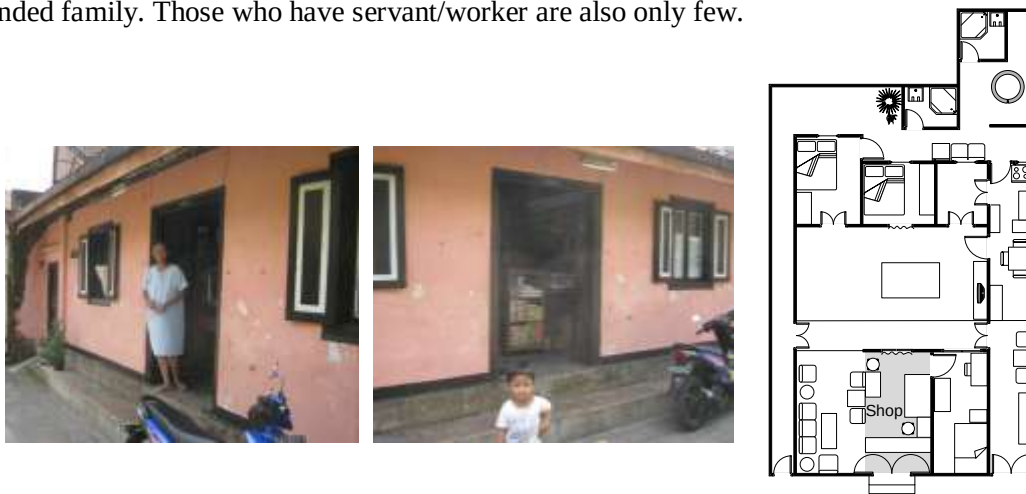
Figure 2.3. One of the Observed Javanese Shop houses
