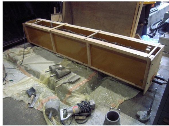
(c) Formwork for SF30-10-r30-L
