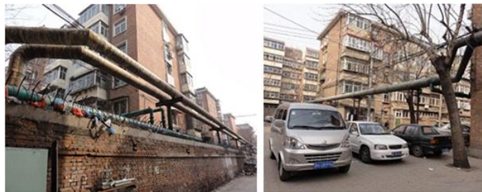
Figure 2-3: Parking and some construction in a residential site built before 1990
