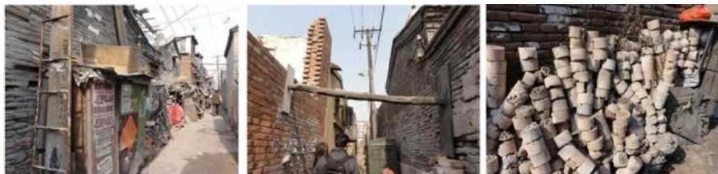
Figure 2-4: Narrow streets blocked by garbage and obstacles in a residential site built around 1960s
