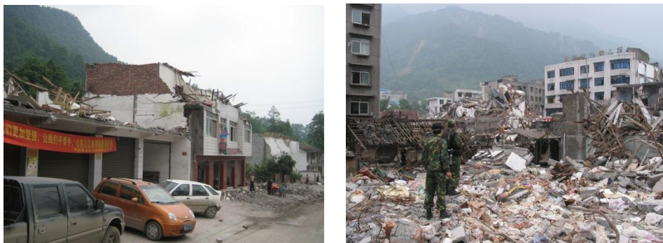
Figure 1-1 Collapse due to the structural failure in the 2008 Sichuan earthquake
