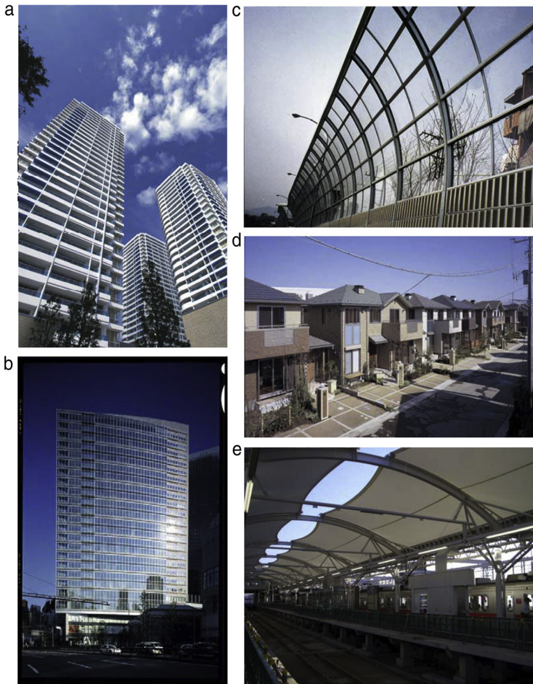
Figure 8 Application of self-cleaning exterior building materials. (a) Picture of the MM Towers, in Yokohama, coated with self-cleaning tiles (courtesy of TOTO). (b) Picture of the Matsushita Denso building covered with self-cleaning glass (courtesy of Nippon Sheet Glass). (c) Picture of the self-cleaning sound-proof wall (courtesy of Sekisui). (d) Eco-life-type houses using self-cleaning tiles and glass (courtesy of PanaHome). (e) Self-cleaning roof of a train station in Motosumiyoshi (courtesy of Taiyo Kogyo).
