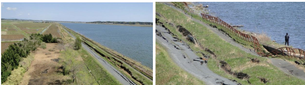
Figure 1.8. Views of slumped Hinuma River Levee and cracks induced by liquefaction (GEER, 2011).
