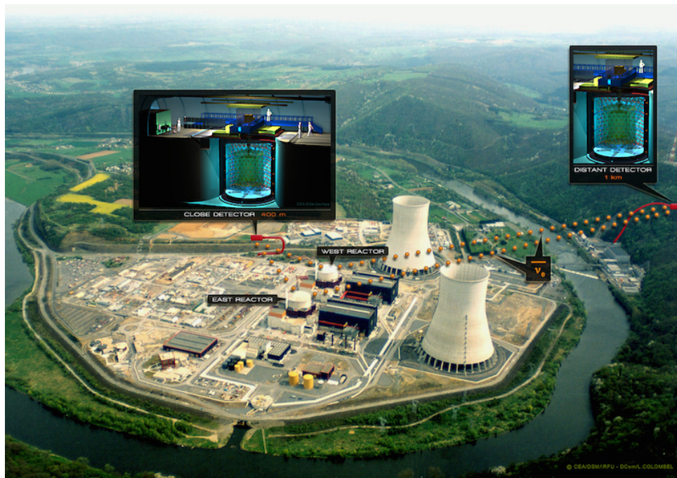
Figure 3.2: A picture of the Chooz reactor complex. The locations of the two reactors as well as the two detectors are shown.
