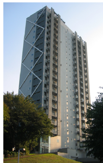
Figure 1. External appearance of 20-story high-rise seismic isolated steel building ( J2-building )
