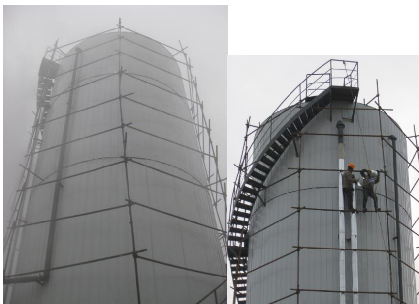
Figure 3.5 The EGSB reactor
