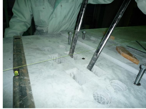
(b) Adjustment of pre-cast deck
