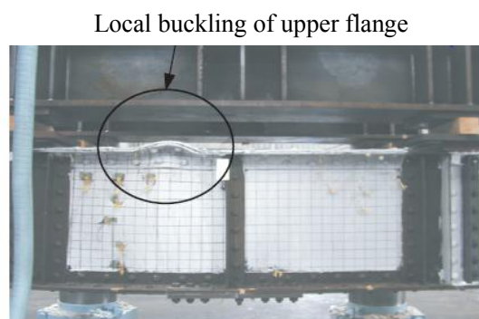
Fig. 1-6 Local buckling of upper flange 12)
