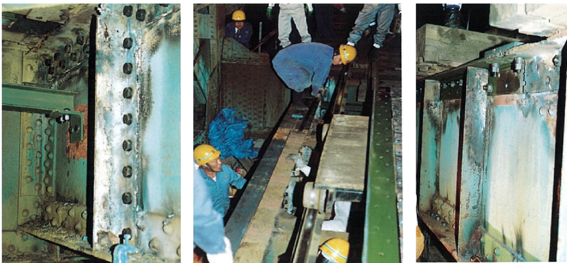
(a) Replacement of rivets to high-strength bolts
