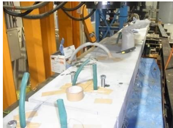
(c) Deck settlement and mortar filling
