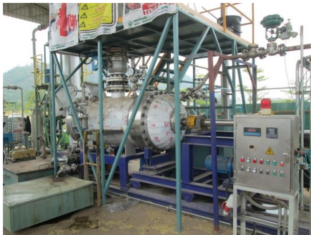
Figure 2-5 Hydrothermal pilot plant (Courtesy of SCG)
