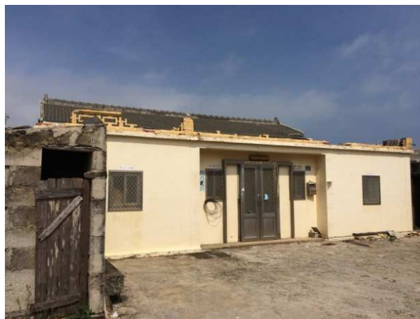
Figure 3.15 GE222 site investigation 2
