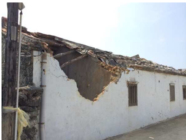
Figure 3.14 GE222 site investigation 1
