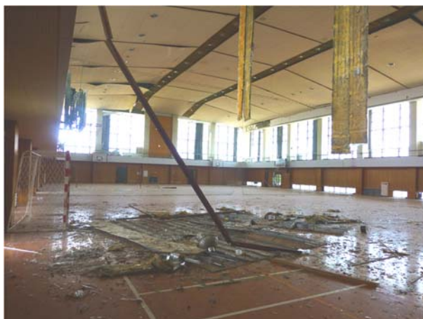
Photo 1 Collapse of Suspended Ceiling in Gymnasium during Kumamoto Earthquake
