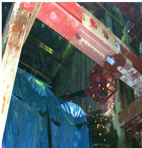
写真 3.23 溶接火花の飛散状況
