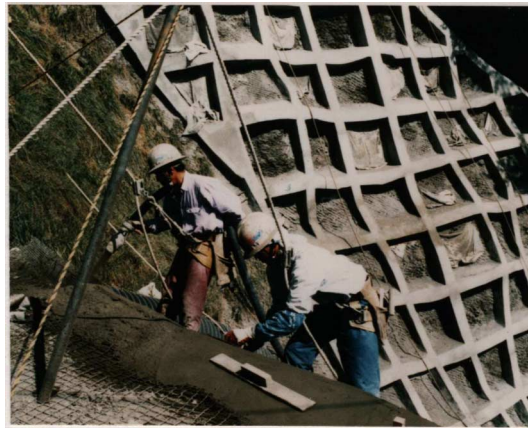
Fig. 2.31: Workers on inclined construction site.
