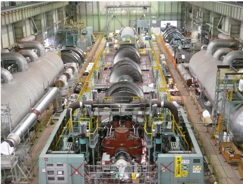
Fig.1.1 Birds-eye view of large power nuclear steam turbine and moisture separator reheaters
