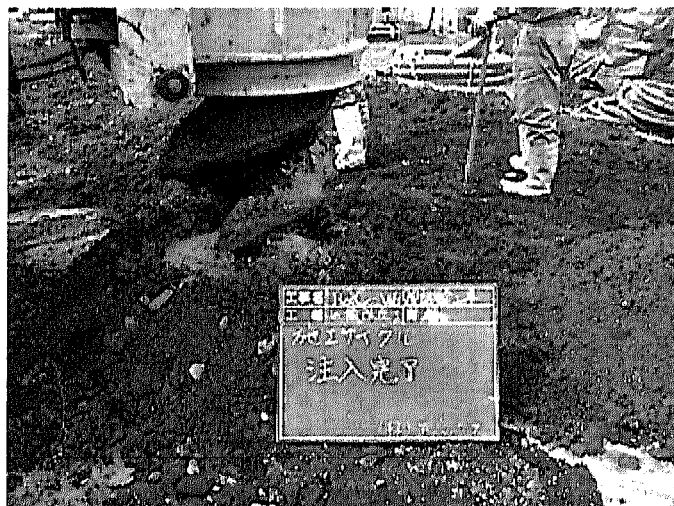
Figure 6.26 Injection of the EPS beads modified cement improvement slurry (completion)
