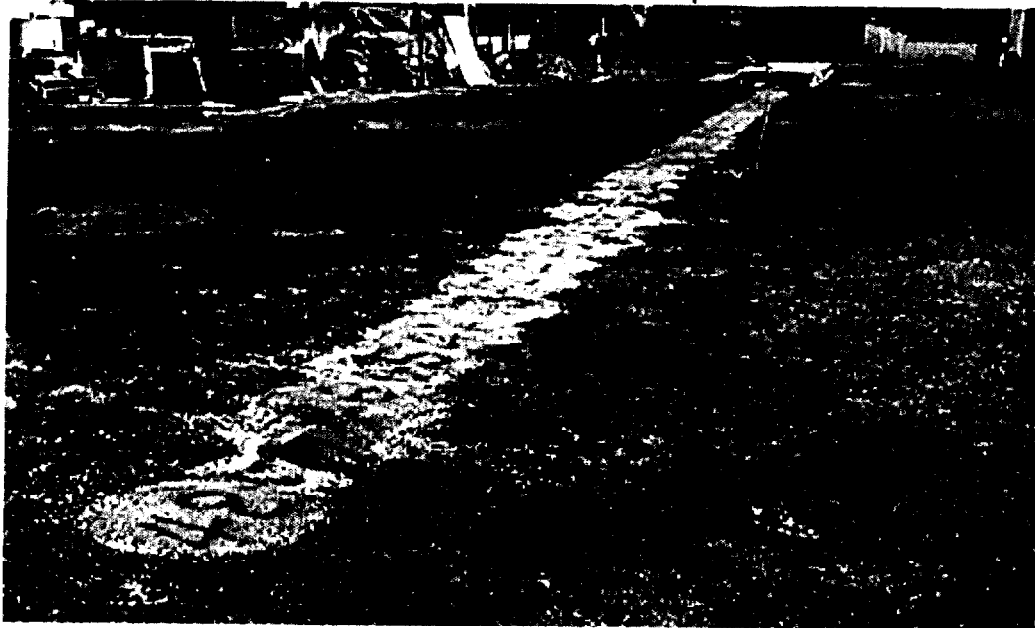
Figure 6.28 Completion condition of constructed wave barrier
