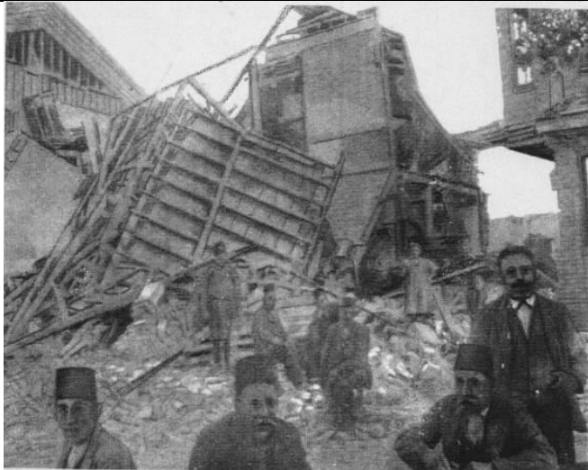
(e) Collapsed buildings at Sarkoy (Sadi, 1912).
