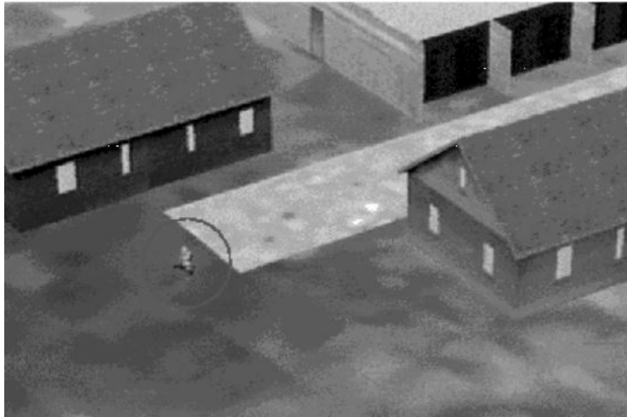
Figure 1.6: Video surveillance and monitoring system
