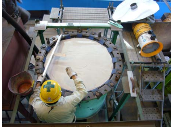
Photo 2.10 Adjustment of surface level
