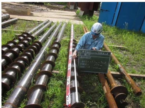
Photo 5.1 Continuous helical pile
