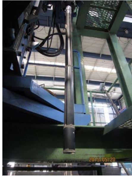
Photo 4.2 Straight sided pile
