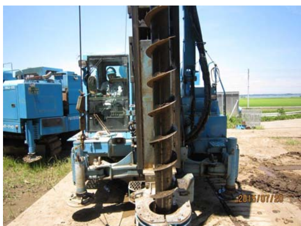
Photo 5.3 Continuous helical pile
