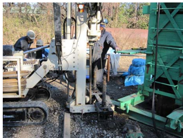
Photo 3.2 Cone penetration test
