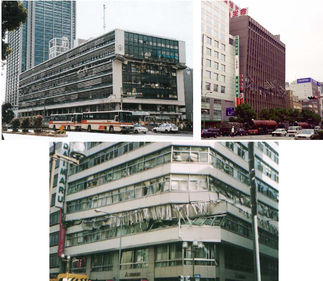
Fig 1.3 Mid-level collapse observed in Great Hanshin earthquake 1995
