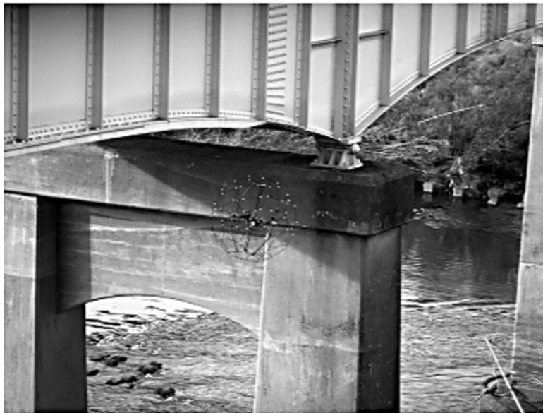
Figure 1.5 Application of UAV for inspection [59]
