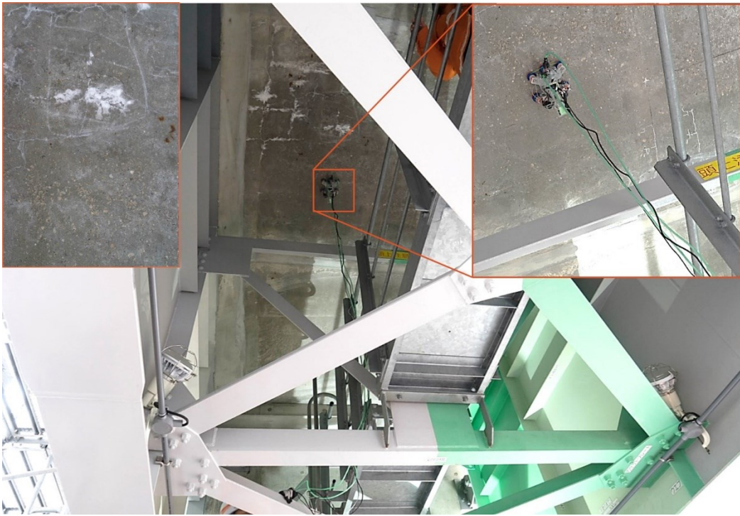
Figure 2.25 Performance test of robotic movement on the trial bridge
