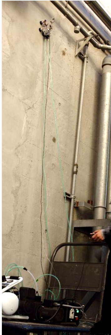
Figure 2.22 Inspection robot during a performance test of robotic movement on an outside concrete wall
