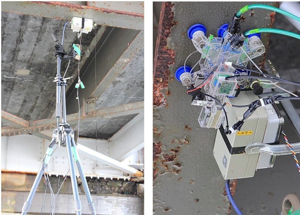
Figure 3.16 Measurement conditions when obtaining bridge vibration
