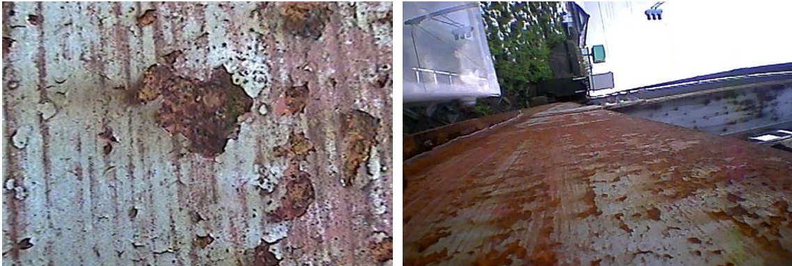
Figure 3.4 Images from both the visual inspection camera and surrounding camera
