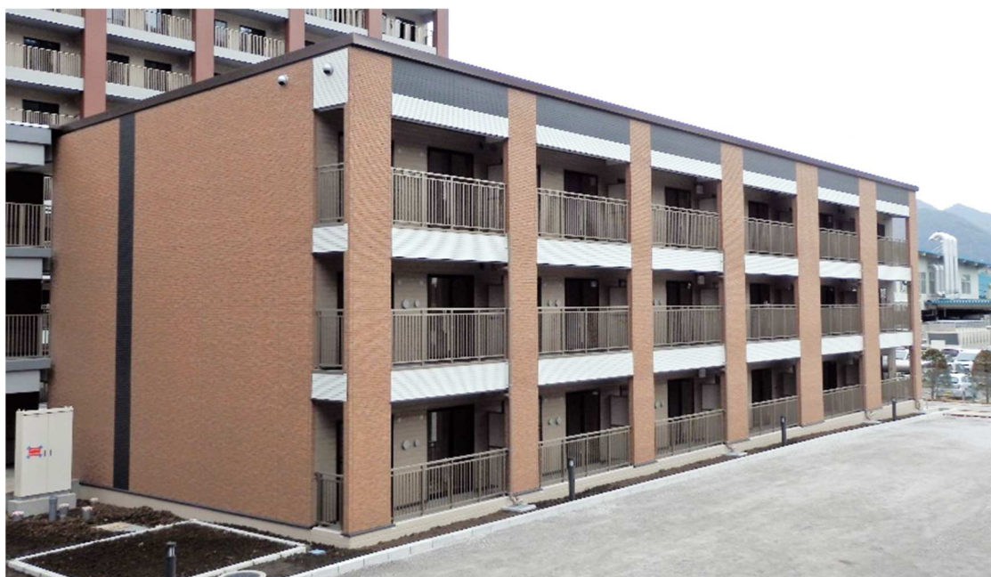
Fig.1.3 Reconstructed residential house after Tohoku earthquake
