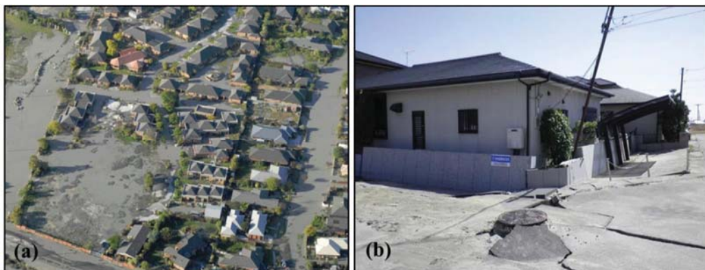
Figure 4.15. (a) Liquefaction damages in 2011 Christchurch earthquake, (b) Liquefaction damages in 2011 Tohoku earthquake (Towhata, 2011).
