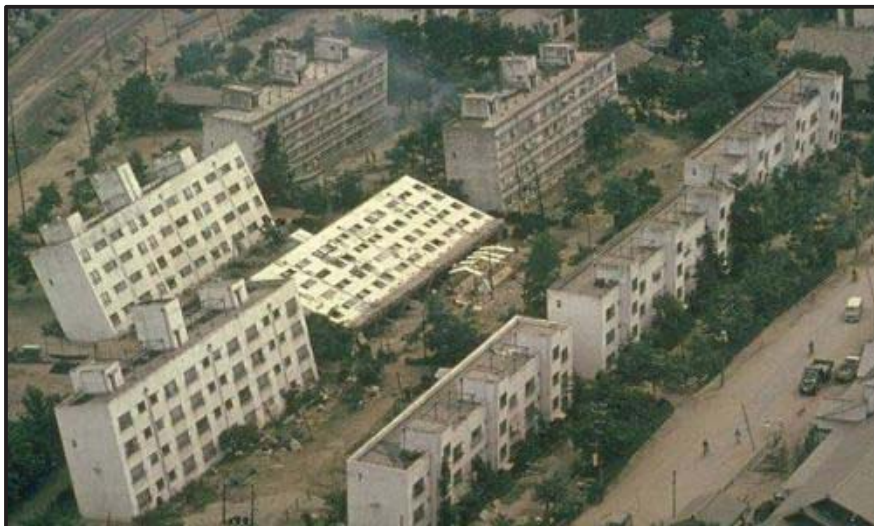
Figure 4.13. Buildings overturning due to liquefaction during 1964 Niigata earthquake.
