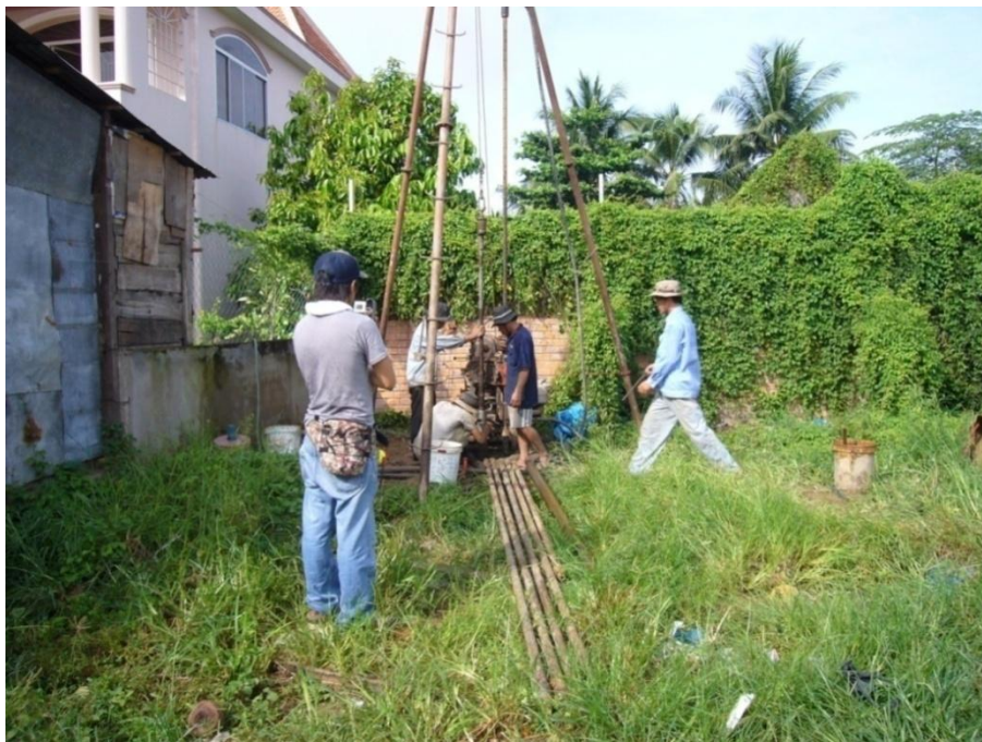
(c) Boring machine was working at Vinhlong site in Vinhlong province MRD.
