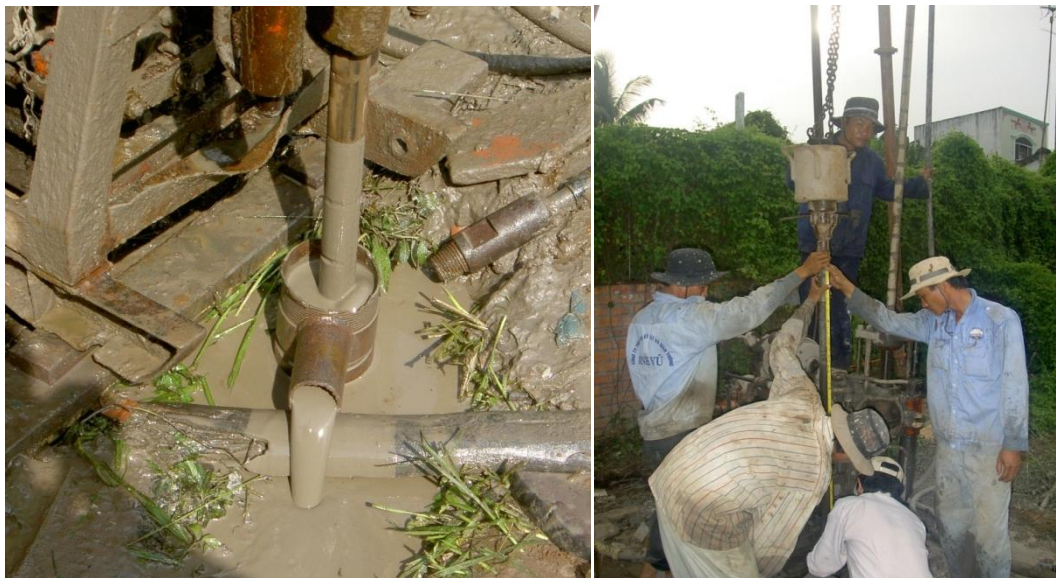
Fig. 3.8. Cleaning sand and remainder soil fragment and checking the depth before conducting SPT test at Vinhlong site in Vinhlong province MRD.
