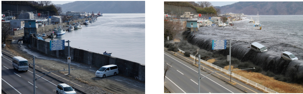
Fig. 1.8 Tohoku Tsunami wave overflows barrier in Miyako, Iwate Prefecture, Japan 2011 (Credit: Reuters)
