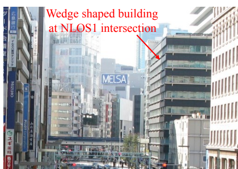
(a) Wedge shaped building at NLOS1.
