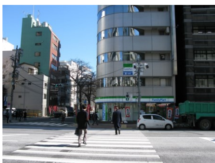
(c) Chamfered shaped building at NLOS3.
