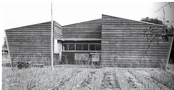
Fig 3. 21 House O, Masako Hayashi, 1951. GCS Diagram. A house for a mother and four children. Top left: view of the kitchen towards the living room. Bottom: West view window kitchen. Photographs from Shinkenchiku 1952
