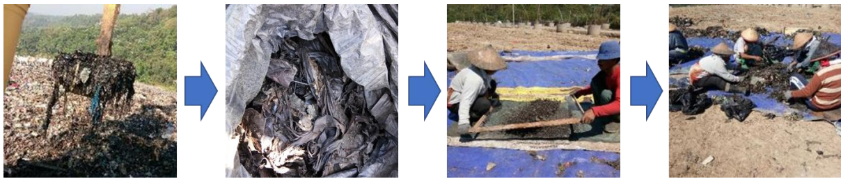
Figure 3.3 Excavation process in Jatibarang Landfill
