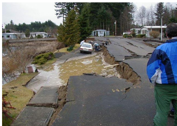
Fig. 1.6. Soil liquefaction and lateral spreading in Tumwater, WA after the 2001 Nisqually Earthquake (Courtesy of UW College of Engineering, USA)
