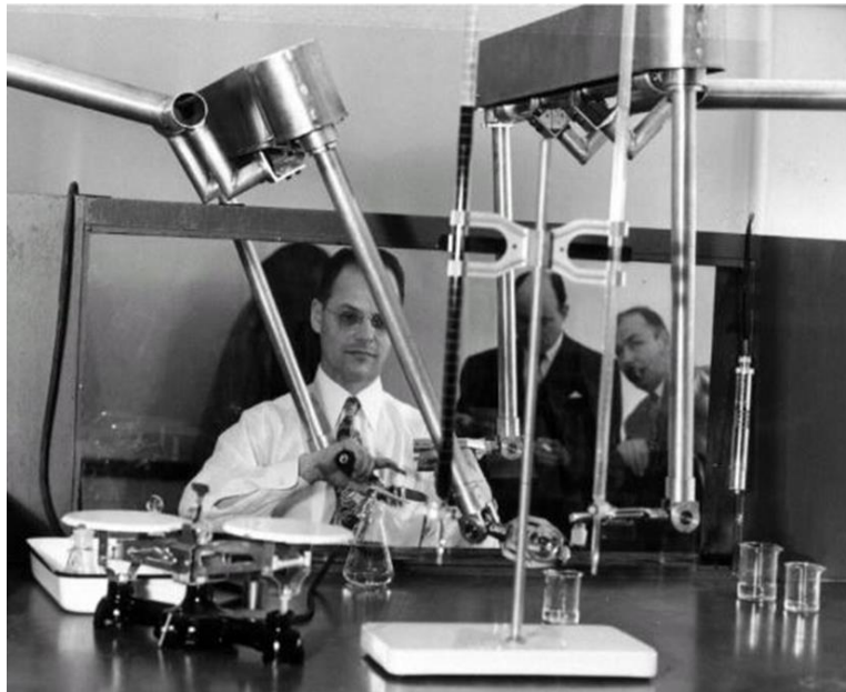
Fig. 1.1 The first master-slave manipulator “model M1” [1].
