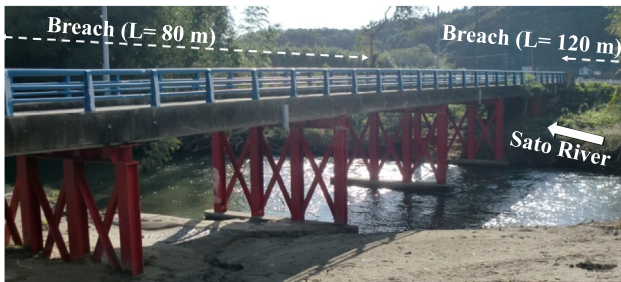
Fig. 31. Akasu Bridge constructed across Sato River.
