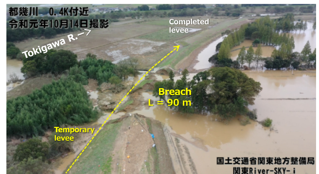
Fig. 7. Breach at 0.4 k on right levee of Tokigawa River. The drone image was obtained from the database maintained by the Ministry of Land, Infrastructure, Transport and Tourism, Japan ( https://www.ktr.mlit.go.jp/bousai/index00000051.html ).
