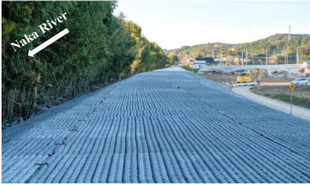
Fig. 18. Temporary restoration works of left levee at 40.0 k of Naka River.
