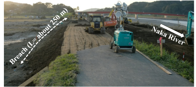
Fig. 20. Temporary restoration works of right levee at 41.2 k of Naka River.
