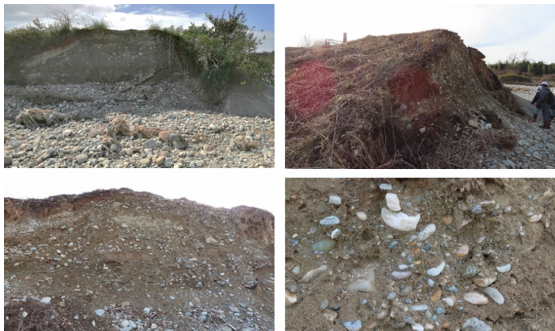
Fig. 25. Damage to levee at breach point. The embankment contains many boulders along with the soil. The embankment was presumably constructed from the surrounding sediment (Photos taken by Unno on December 2, 2019).
