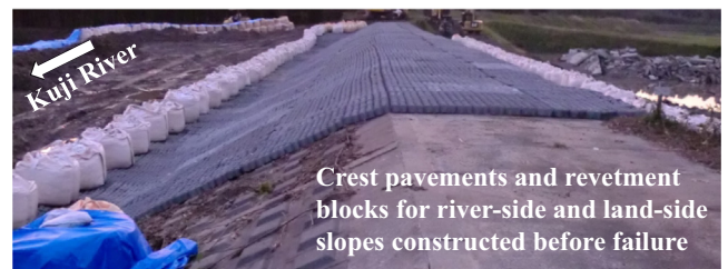
Fig. 28. Crest pavements and revetment blocks for river-side and land-side slopes constructed before failure at 34.0 k of the Kuji River.
