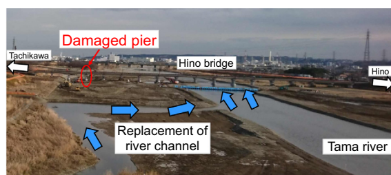
Fig. 42. River channel replacement for restoration work of Hino Bridge.
