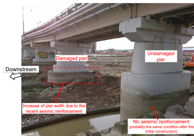
Fig. 44. Damaged pier during the restoration work (from downstream).
