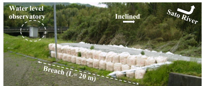
Fig. 34. Temporary restoration works of right levee of Sato River at Point A in Fig. 29.
