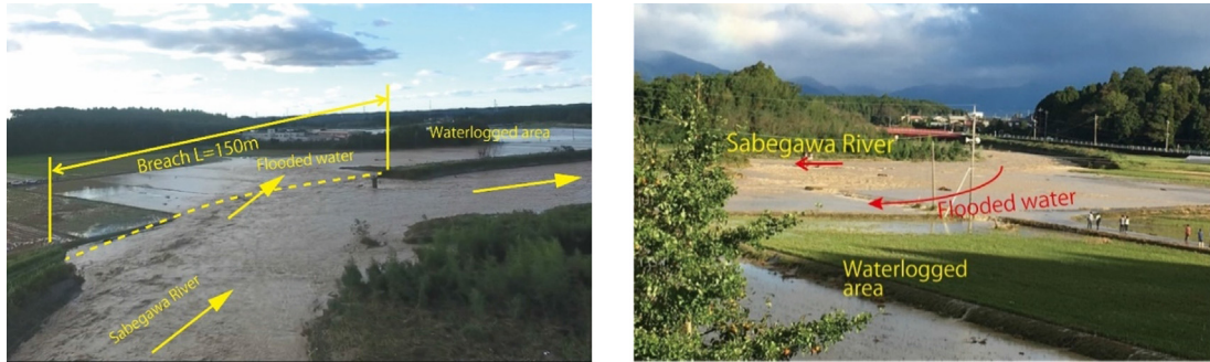
Fig. 22. Breached point on Sabigawa River (in Naka River system) in Kita-owagu area, Otawara City, Tochigi Prefecture. Left photo: View from upstream side, Right photo: View from left levee (Photos provided by Tochigi Prefectural Office with English translation).
