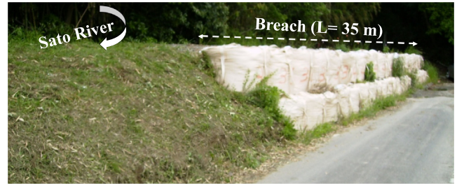
Fig. 33. Temporary restoration works of left levee of Sato River at Point B in Fig. 29.
