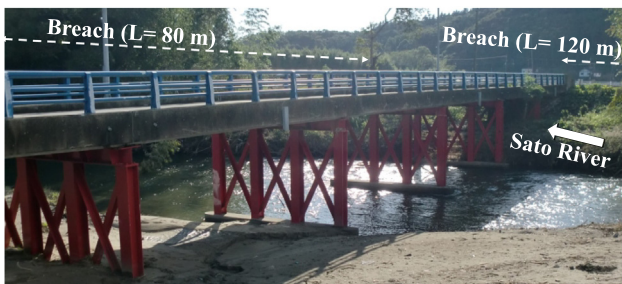
Fig. 31. Akasu Bridge constructed across Sato River.
