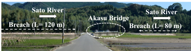
Fig. 30. Temporary restoration works of right levee of Sato River at Point C in Fig. 29 (near Akasu Bridge).
