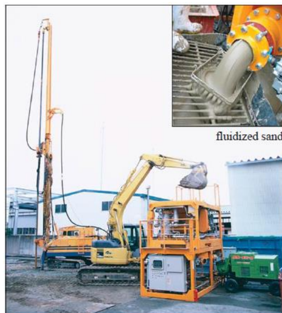
Figure 3.2.1 SAVE-SP machine and mixing plant (Kitazume et al. , 2016).
