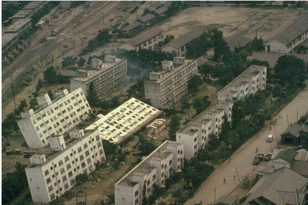
Figure 2.1.1 Collapse of buildings due to loss of bearing capacity during 1964 Niigata earthquake (University of Washington, 2000)
