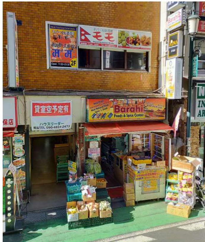
Fig 3.4 Barahi grocery shop with associated Nepalese restaurant on the second floor in ShinOkubo
