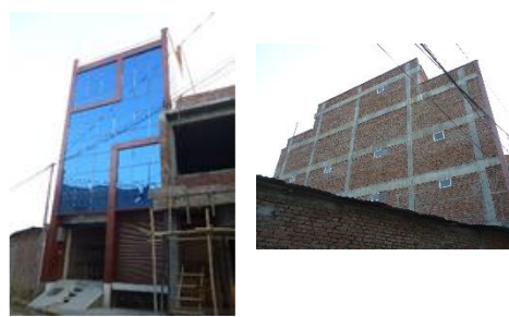
Picture 1 Overview of target building
