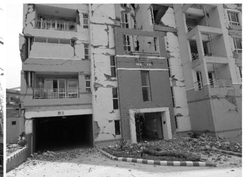
Photo 2 Out-of-plane failure of infill walls in the 2015 Nepal earthquake
