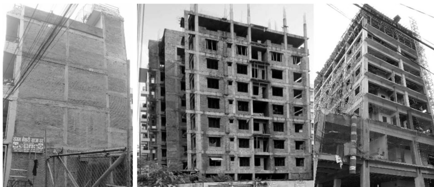
a) Nepal b) Bangladesh c) Indonesia Photo 1 RC buildings with brick masonry infill walls
