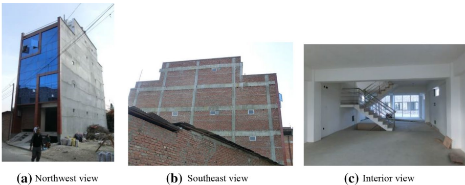
Fig. 3 Overview of the study building
