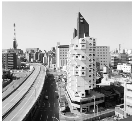
Fig.1. Nakagin Capsule Tower, Kisho Kurokawa architects and associates, 1972
