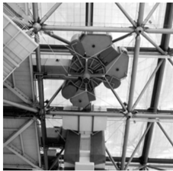
Fig. 53. Few monofunctional units added together to the main core in Capsule house, 1970, Kisho Kurokawa
