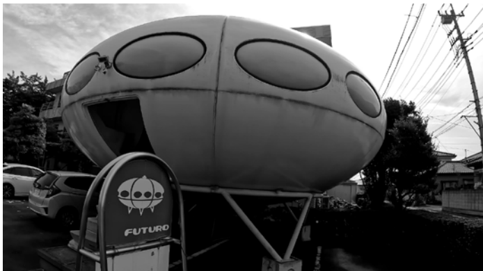
Fig.3. Fiberglass-reinforced polyester plastic panels are connected and sealed by thick layer of silicon. The blurred windows are for bedroom, bathroom unit and other technical spaces.
