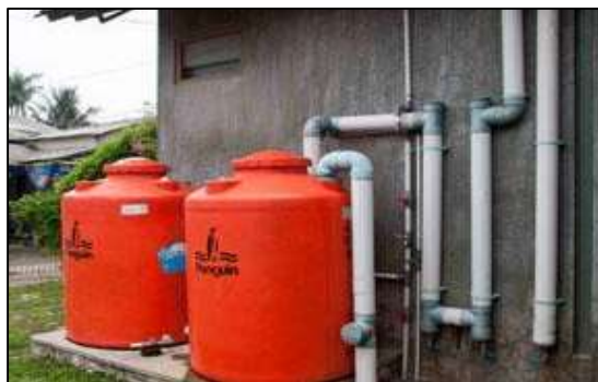
Figure 12: Rainwater harvesting in the study area
