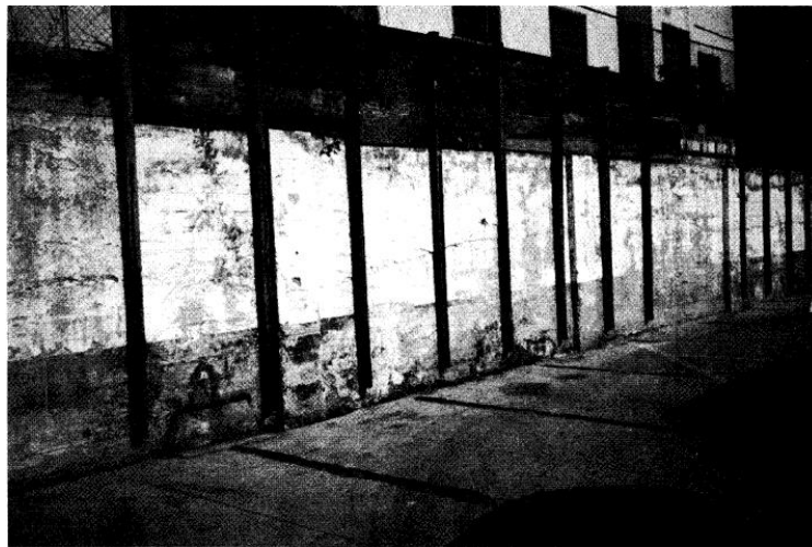
Figure 2.13: Cantilever retaining wall in case study 1.
