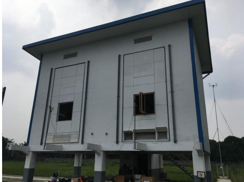
Fig. 3.1. Experimental building in Tangerang, Indonesia
