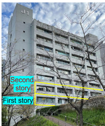
Figure 4. Northeast view of study building.
